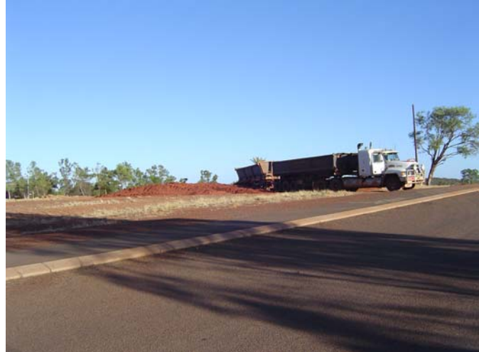
Above: Simon Thomas delivers soil on blocks at Scotia and Walls Streets to begin 3 DHW Houses.
